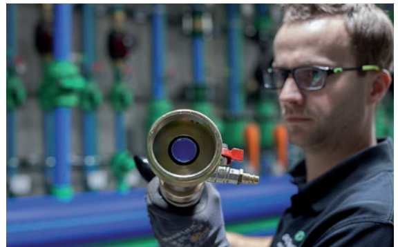
4. After the drilling operation, the tapping tool is removed from the component unit.
